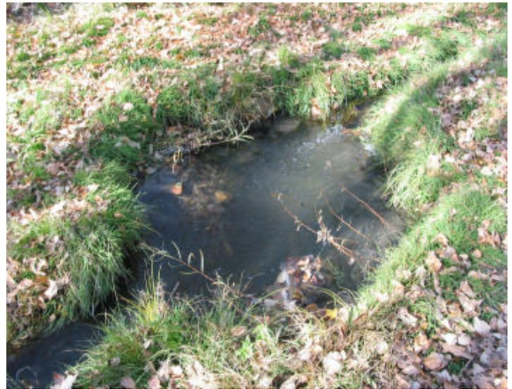
**Photo of a rock v-weir pool, complete with fish cover habitats. The pool habitat was constructed on Millennium Creek this summer.**
